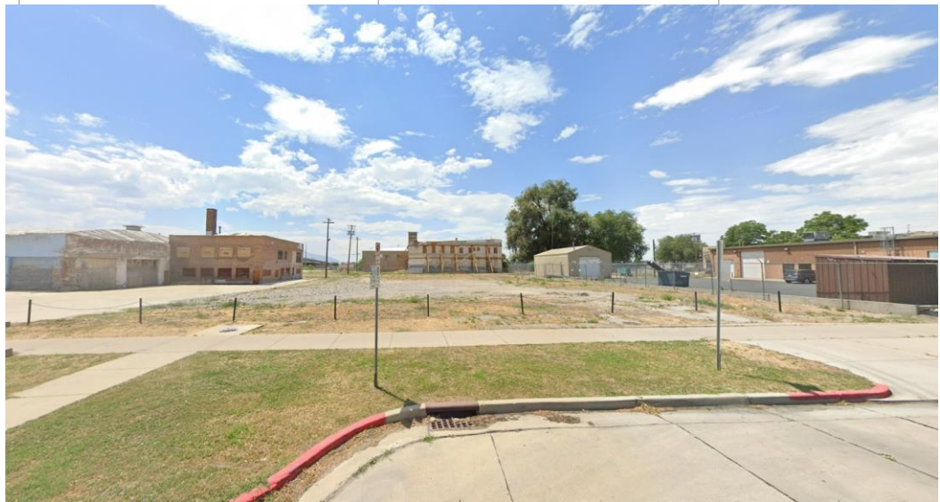
View of site from 500 West with Salt Lake Mattress Company building in distance and 'Blue Warehouse' to the south. State arts and artifacts building can be seen to the far right of the image.
